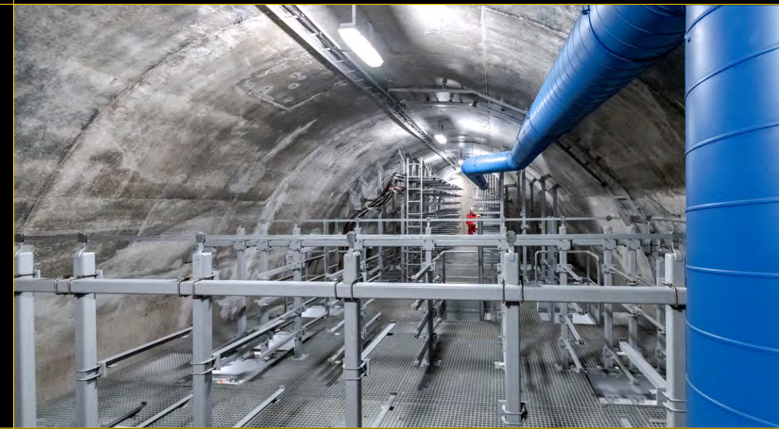
2016 KOLEKTOR HLÁVKŮV MOST V PRAZE 2016 HLÁVKA BRIDGE UNDERGROUND UTILITY TUNNEL
