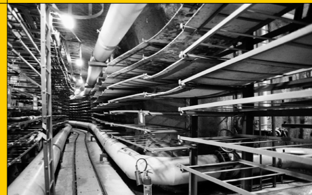
KOLEKTOR CENTRUM I, PRAHA CENTRE I UNDERGROUND UTILITY TUNNEL, PRAGUE
