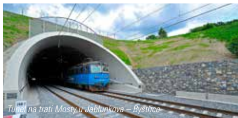
Tunel na trati Mosty u Jablunkova – Bystřice
